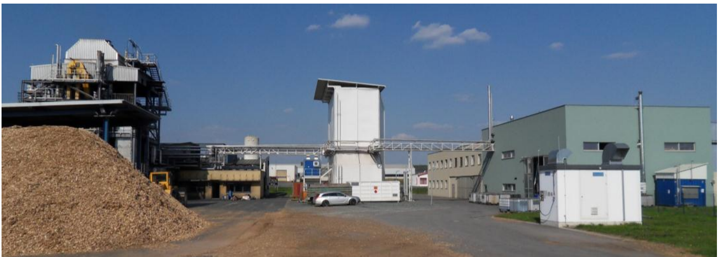
Figure 2: Biomass CHP Güssing with BioSNG demonstration plant and Technikum.
