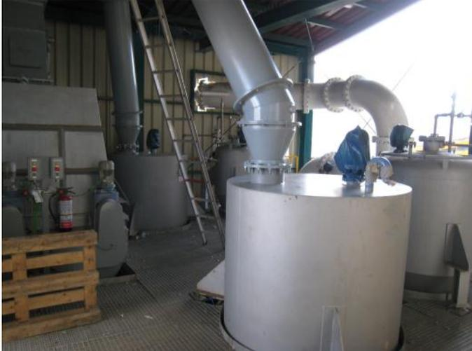
Figure 2: Inert feeding system.
