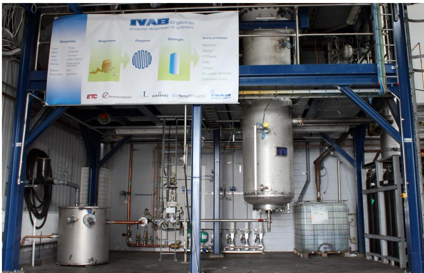
Figure 1: Mounting stand and lower parts of the PEBG installation at ETC. The gasifier vessel containing gasification reactor and cooling quench is seen in the centre of the picture.
